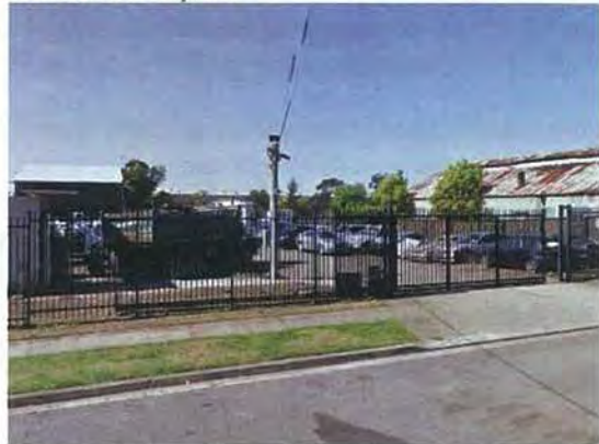
Photo 6: Survey Unit 1 – 26 Shepherd Street, southeast aspect
