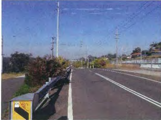
Photo 23: Survey Unit 3 –Powerhouse Rd, southwest aspect
