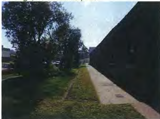
Photo 1: Survey Unit 1 – Shepherd Street frontage, northeast aspect
